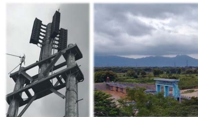
Indonesia: Dam water discharge alert system
